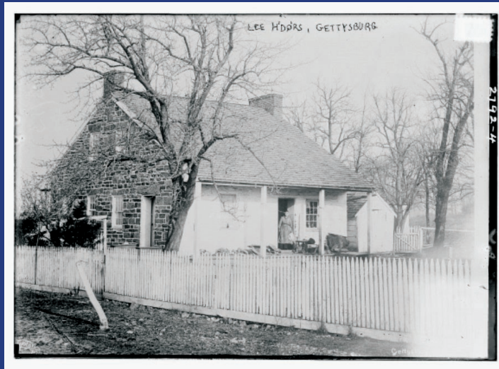
Left: House that served as Robert E. Lee's headquarters at Gettysburg.
